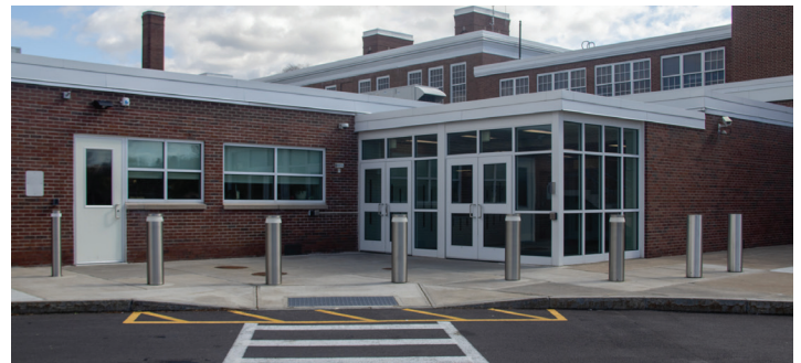
▲ Site Deterrents were successfully installed to prevent automobiles from accessing our glass door entry ways and sidewalk spaces.
